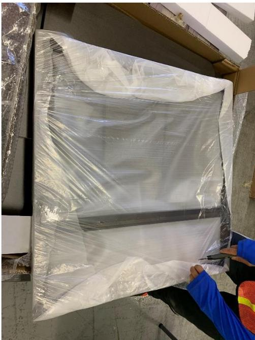
Step 3. Take the left side panel to align it on the groove present on back face of the Cabinet Frame. Ensure the top and bottom of the panel is aligned equally to the edge of the frame. Attach the bracket at top and bottom of the panel with a screw
