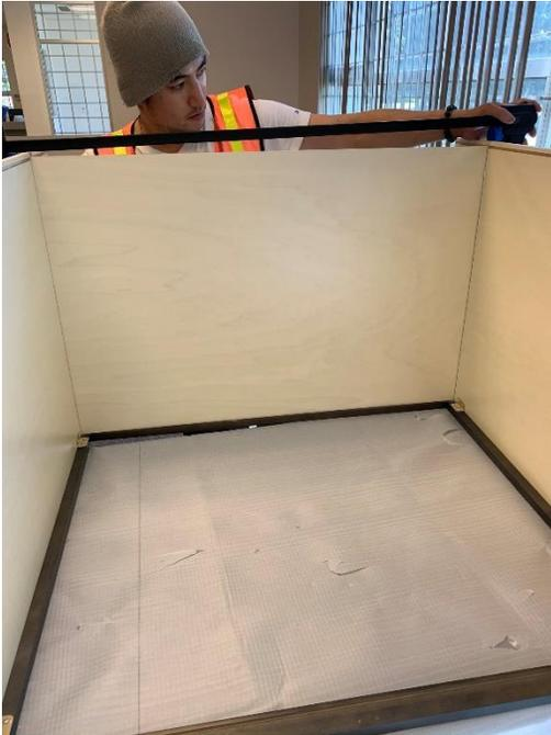
Step 6. Slide the back panel along the groove and ensure it neatly fits along the three edges. Secure the sides from behind with screws and at the bottom with brackets
